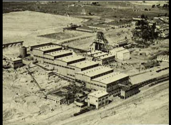
No. 2 Shaft & Concentrator, 1940
