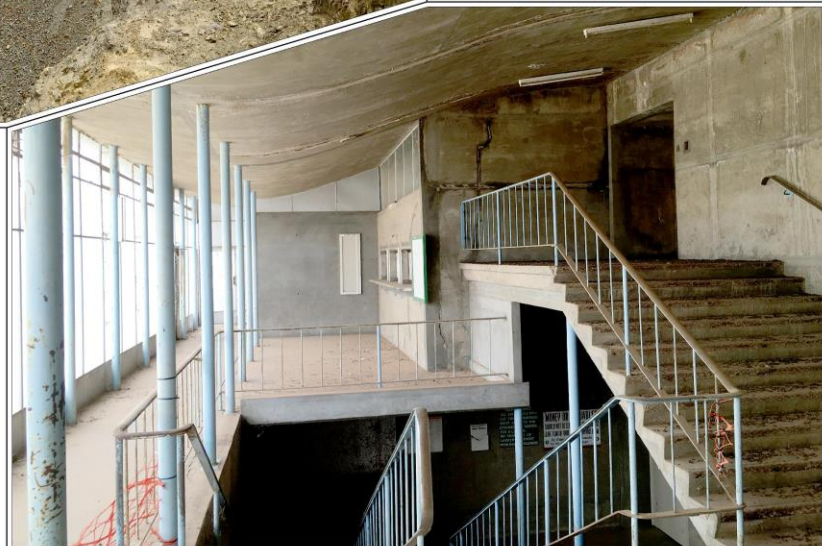
Plate 2.4: Internal view of the North Mine Change House (Ref: A130116_IMG3204)
