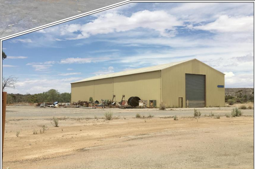
Plate 2.8: External view of the existing store shed (Ref: A130116_IMG_3278)
