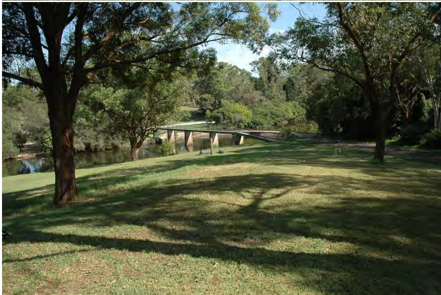
Figure 3.5: View across the northwestern part of the buffer zone towards the Noller Bridge.
