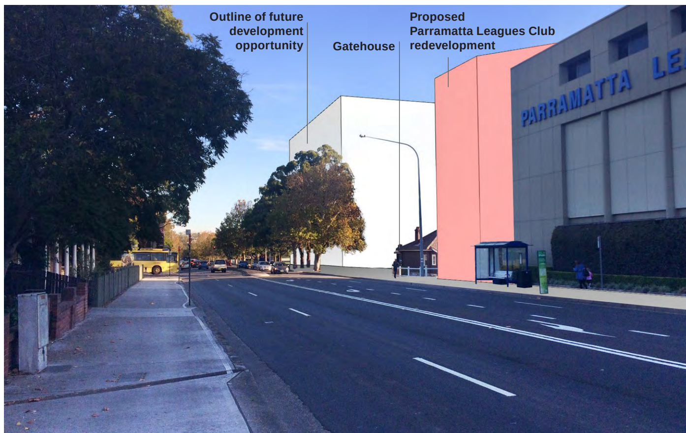
Existing view with the future development opportunity beyond and the Parramatta Leagues Club redevelopment in the foreground
