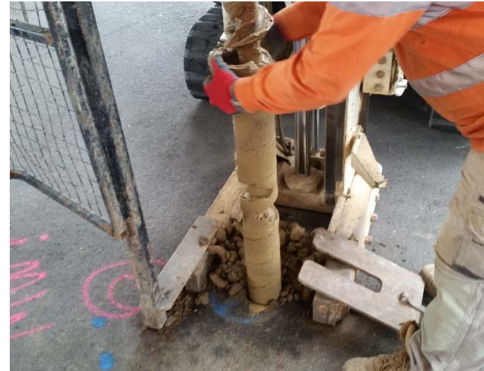
Groundwater encountered at BH47/MW04a location
