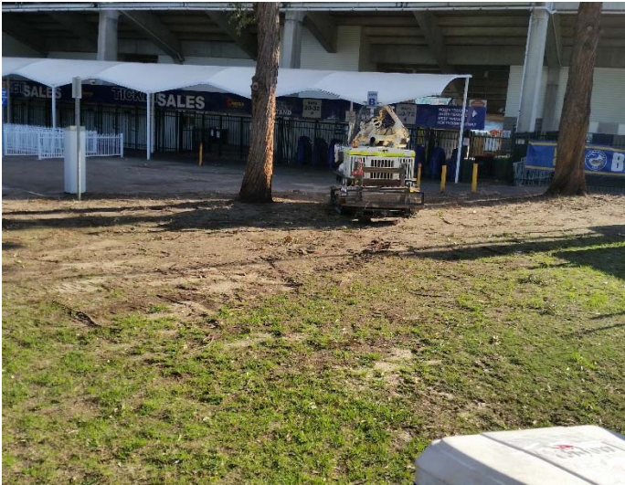
BH20 Location, grassed area near the Eastern forecourt of the stadium.
