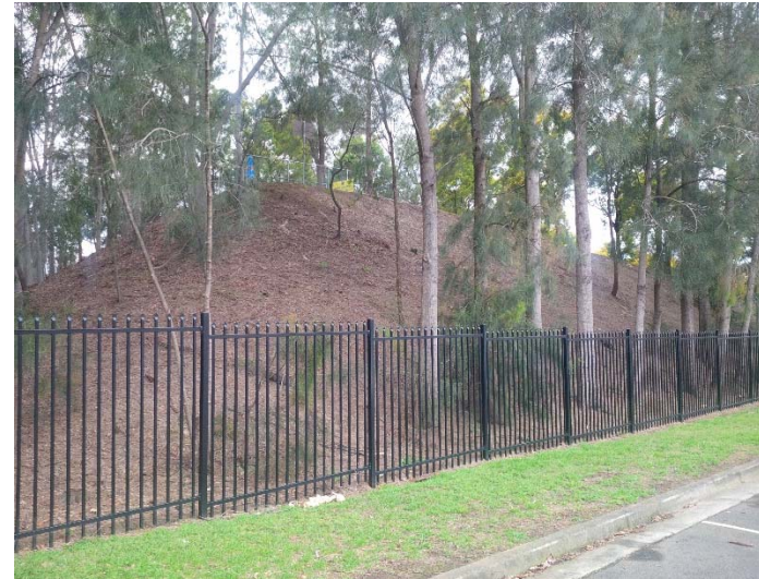
Waterslide Fill Mound within PSC, beyond the Study Area Boundary in the South East of the Site
