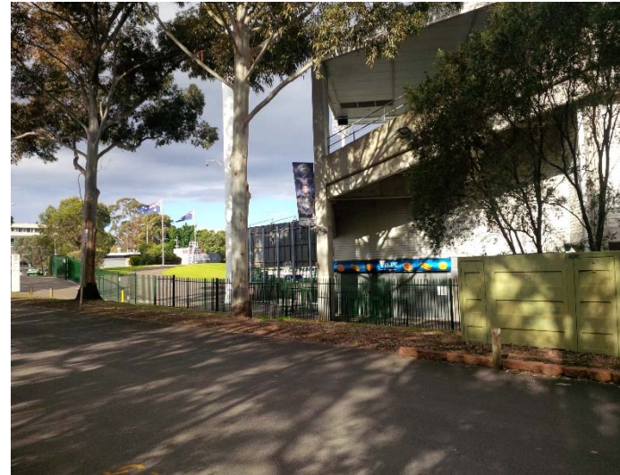
North-west extent of Stadium and access road with electricity substation in the foreground
