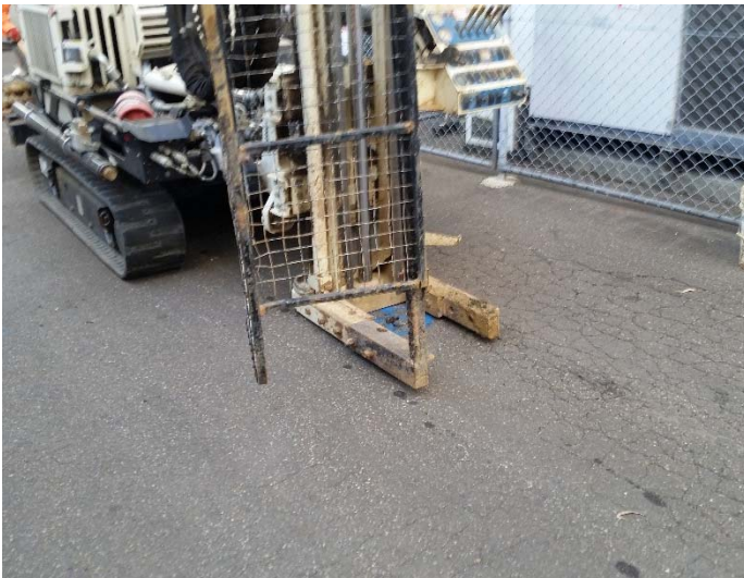
Location of BH49. Eastern area within the stadium.
