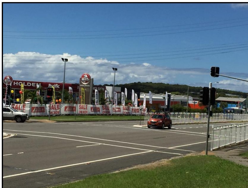
Photo 6 – Commercial Premises on Pacific Highway (looking south east)
