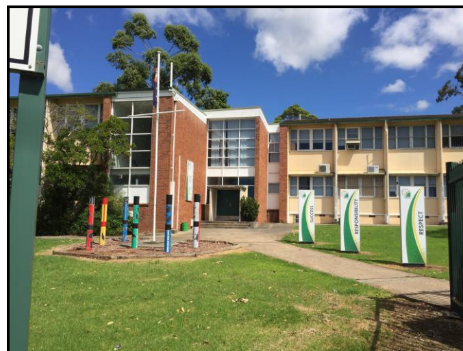
Photo 2 – Administration (looking west)
