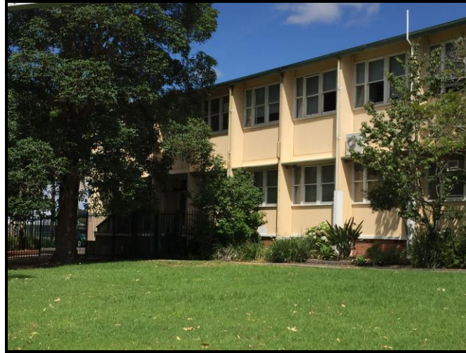
Photo 3 – Existing Classrooms (looking south west)
