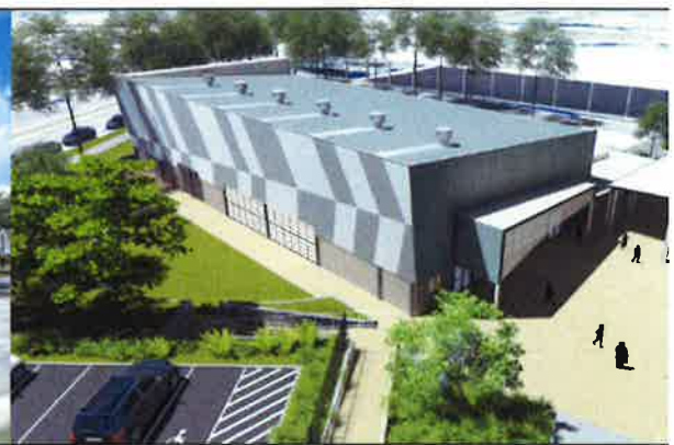
Figure 18 – Southwest aerial view
