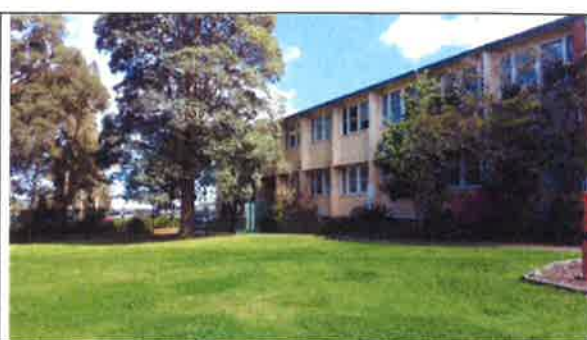
Figure 4 – Existing classrooms (Block E)
