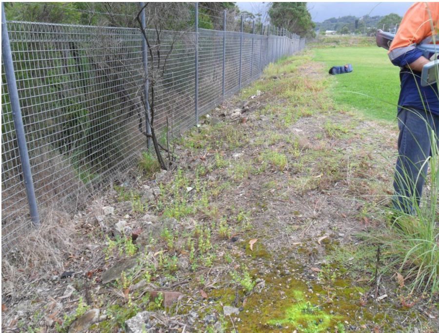
Figure 10: Filling with building rubble on the central-western site boundary, looking north
