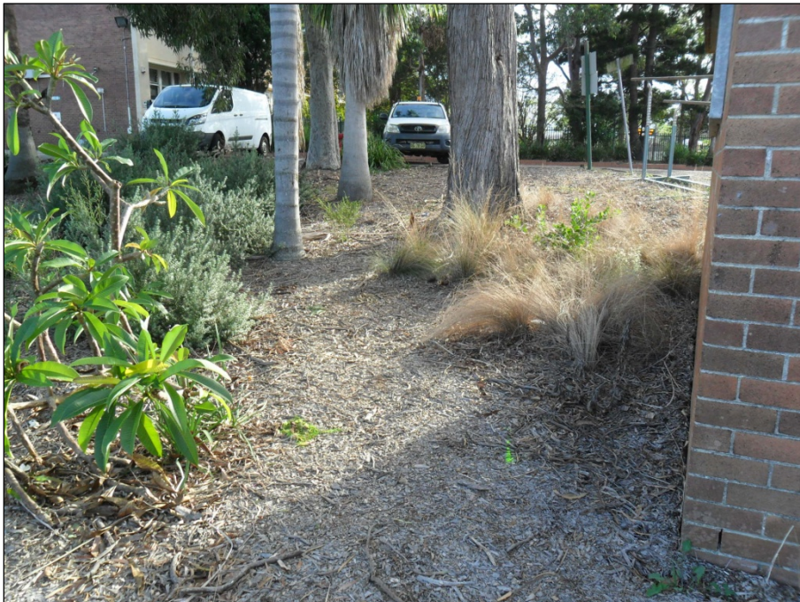
Figure 2: Former substation (brick structure in right of photo)
