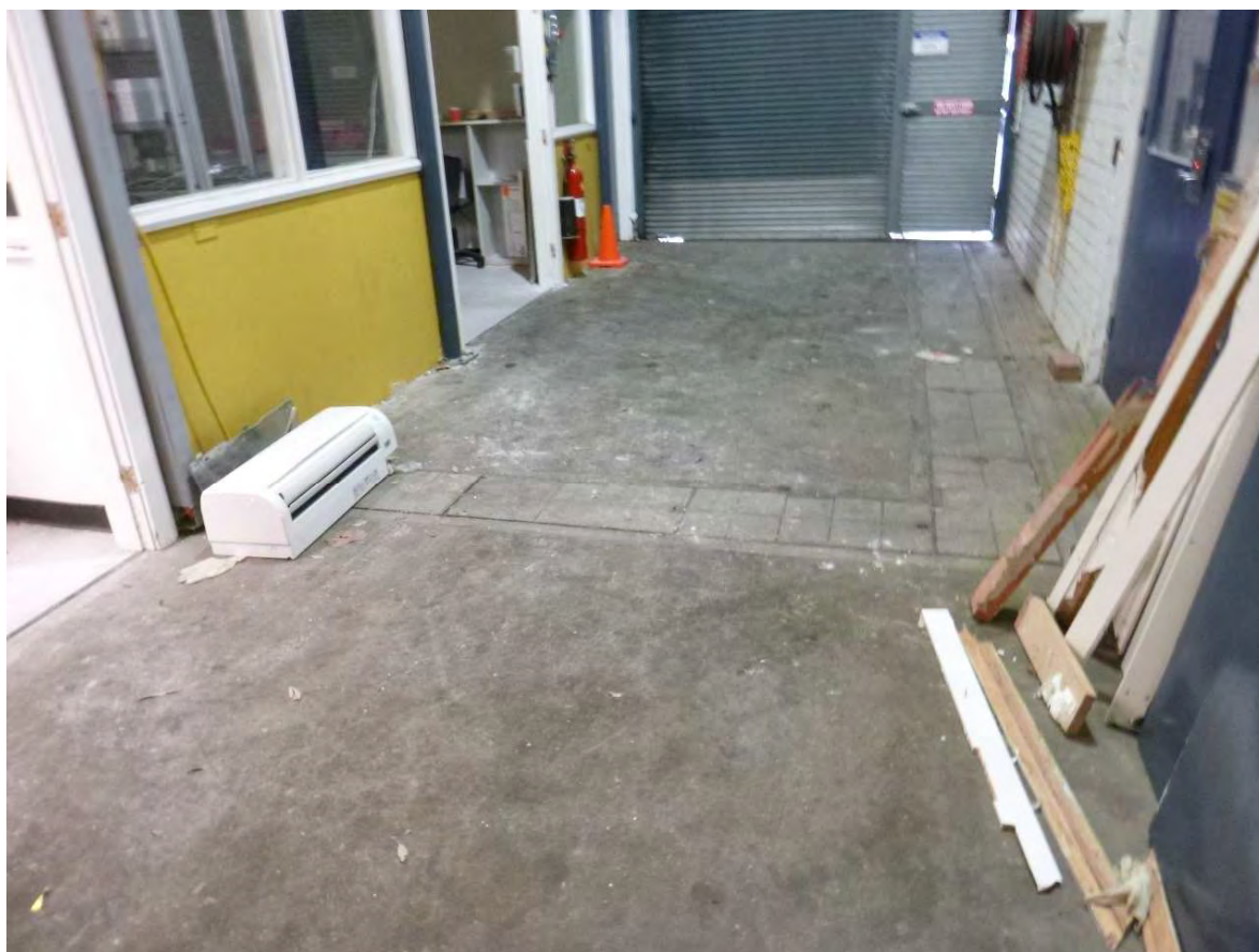
Plate 11: Loading dock area within the ground floor, at the northern end of Metallurgy Process Building (D7)
