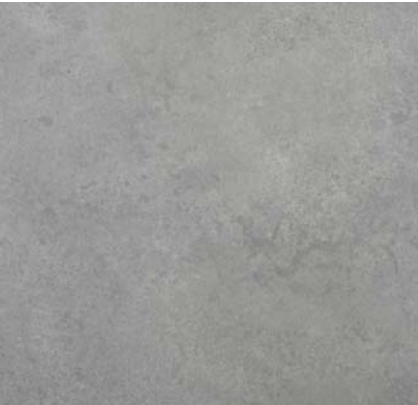
COB SPORTS HALL CONCRETE WITH OXIDE PRECAST BLADE
