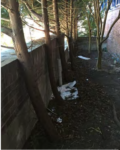
Fig. 19: Depicts Trees 36 in their growing environment pushing against the wall. Source: Austin 11/05/2016
