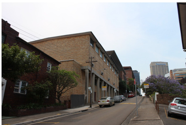
Existing gymnasium on the development site
