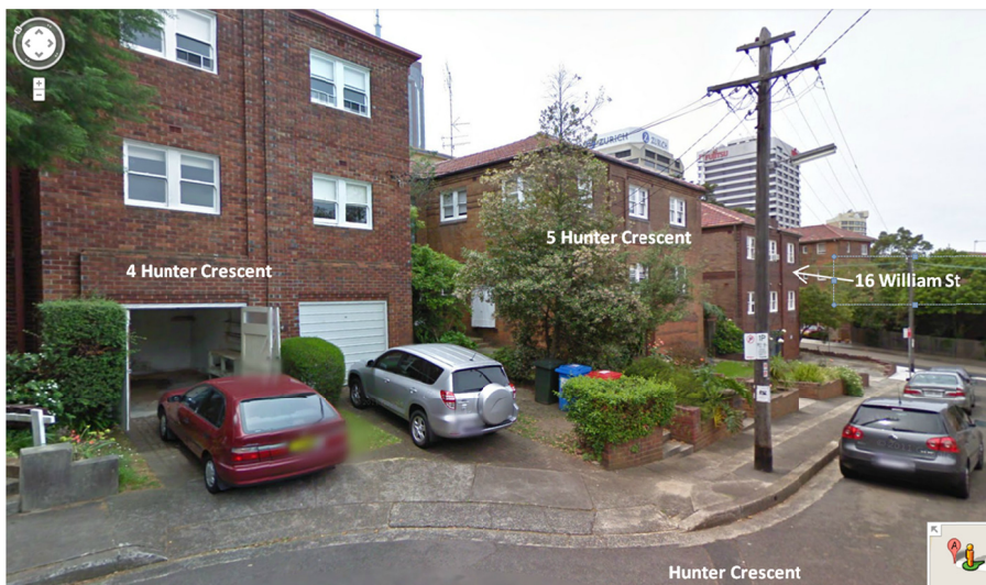
Existing residential flat buildings on Hunter Crescent and William Street
