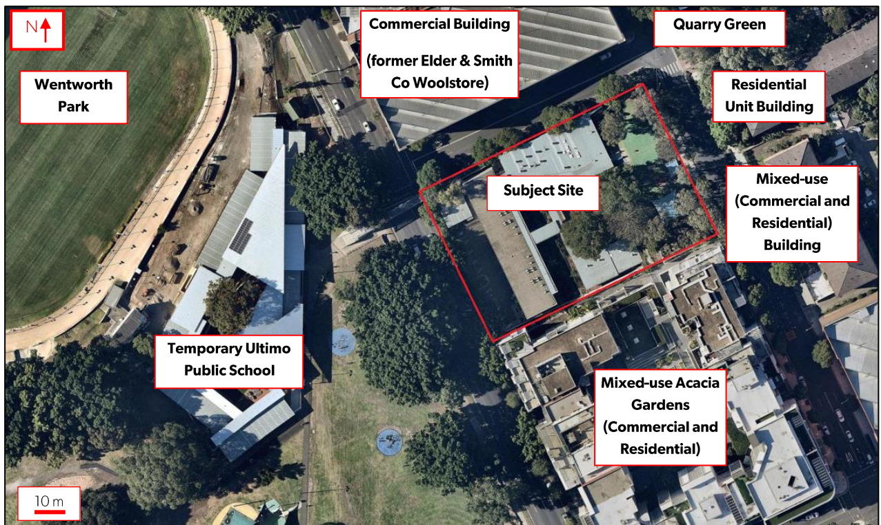
Figure 3 | Surrounding development (Source: Nearmap 2017)
