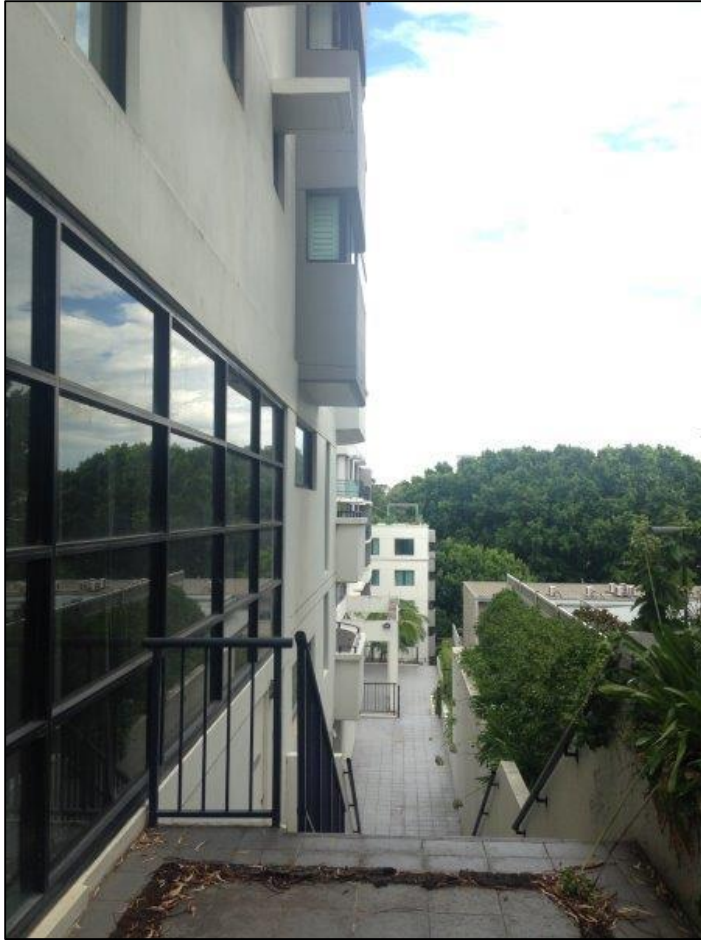
Photo 4 - Existing condition – View from Jones Street looking west along the boundary with neighbouring apartments
