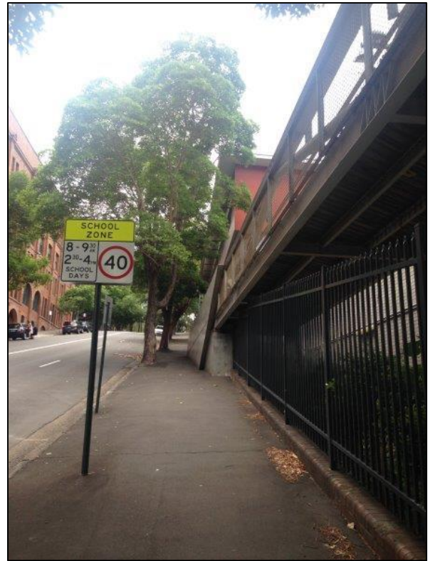
Photo 2 - Existing condition – View looking east on Quarry Street
