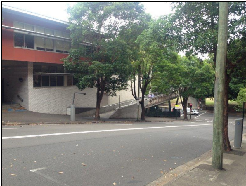
Photo 3 - Existing condition – View looking west on Quarry Street (pedestrian bridge)
