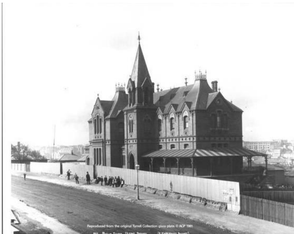
Figure 28 – The original Ultimo Public School (1880-1932), located at a different site on Murray and Pyrmont Streets
