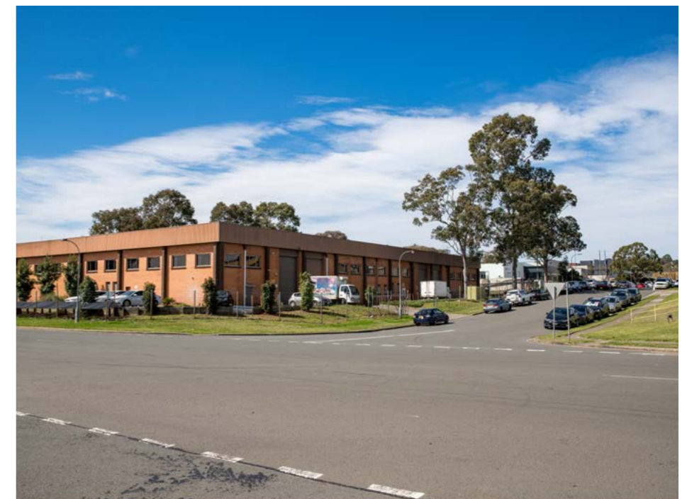
View 18 Detail of 103 Airds Road north of the subject site
