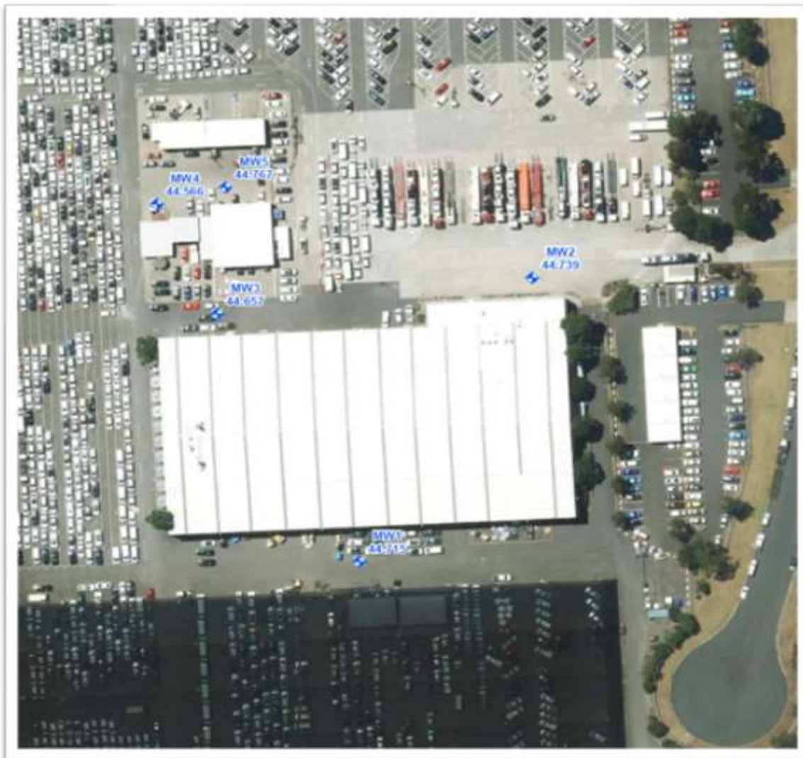
Figure 3: MW01-MW05 Locations located adjacent to the fuel storage and dispensing area.
