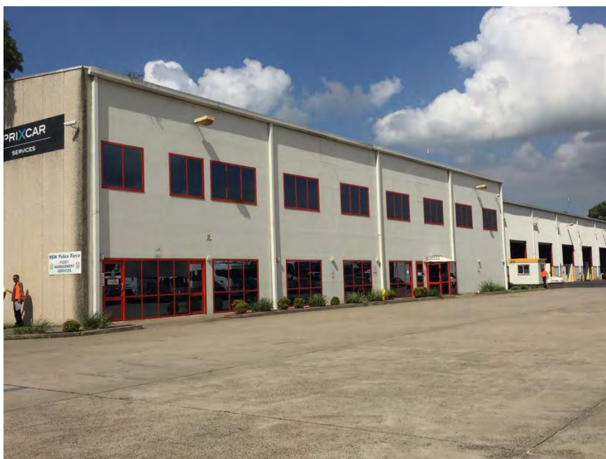
35. The main warehouse building, in the middle of the facility, facing southwest
