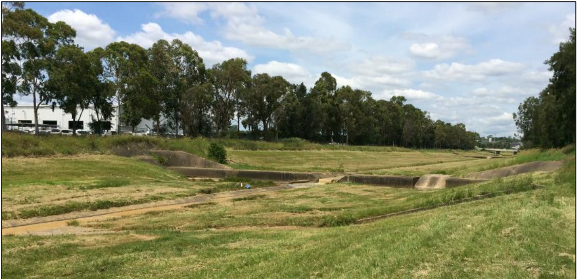
Photo 3: Bow Bowing Creek, one of several drop structures viewing southward (upstream) along the western site boundary.
