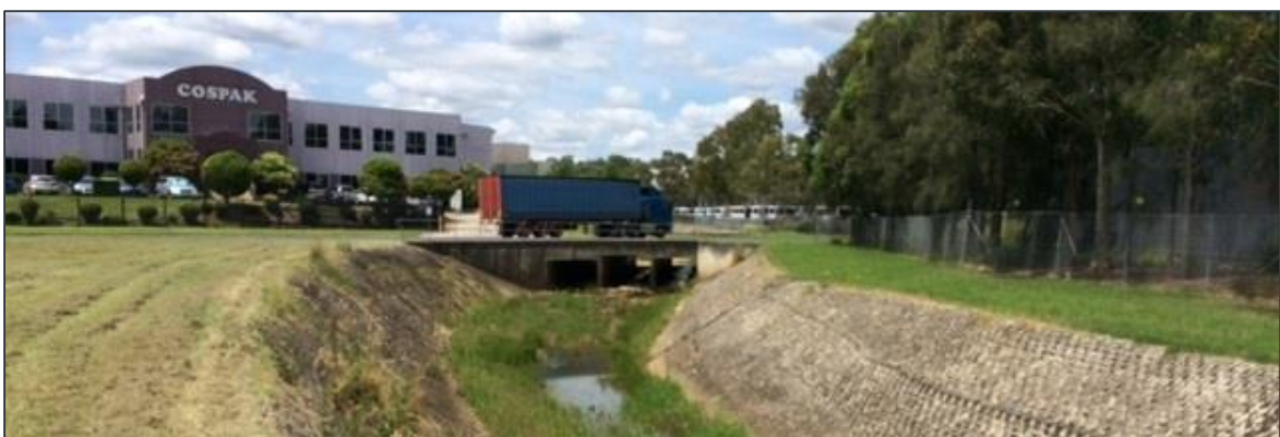
Photo 1: Culverston Road culvert viewing eastward (upstream) along northern site boundary.
