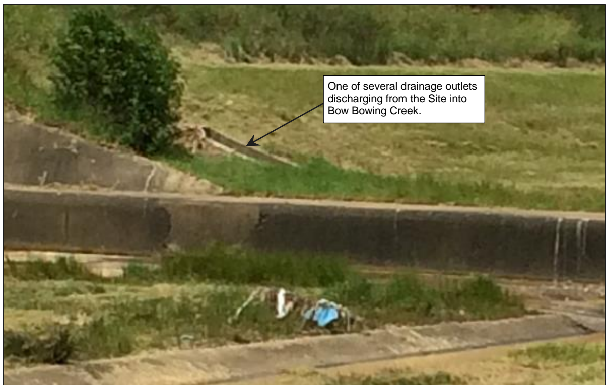
Photo 5: An existing drainage outlet structure on Bow Bowing Creek
