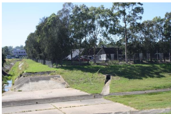
Plate 2: View of drainage canal to north and west of study area
