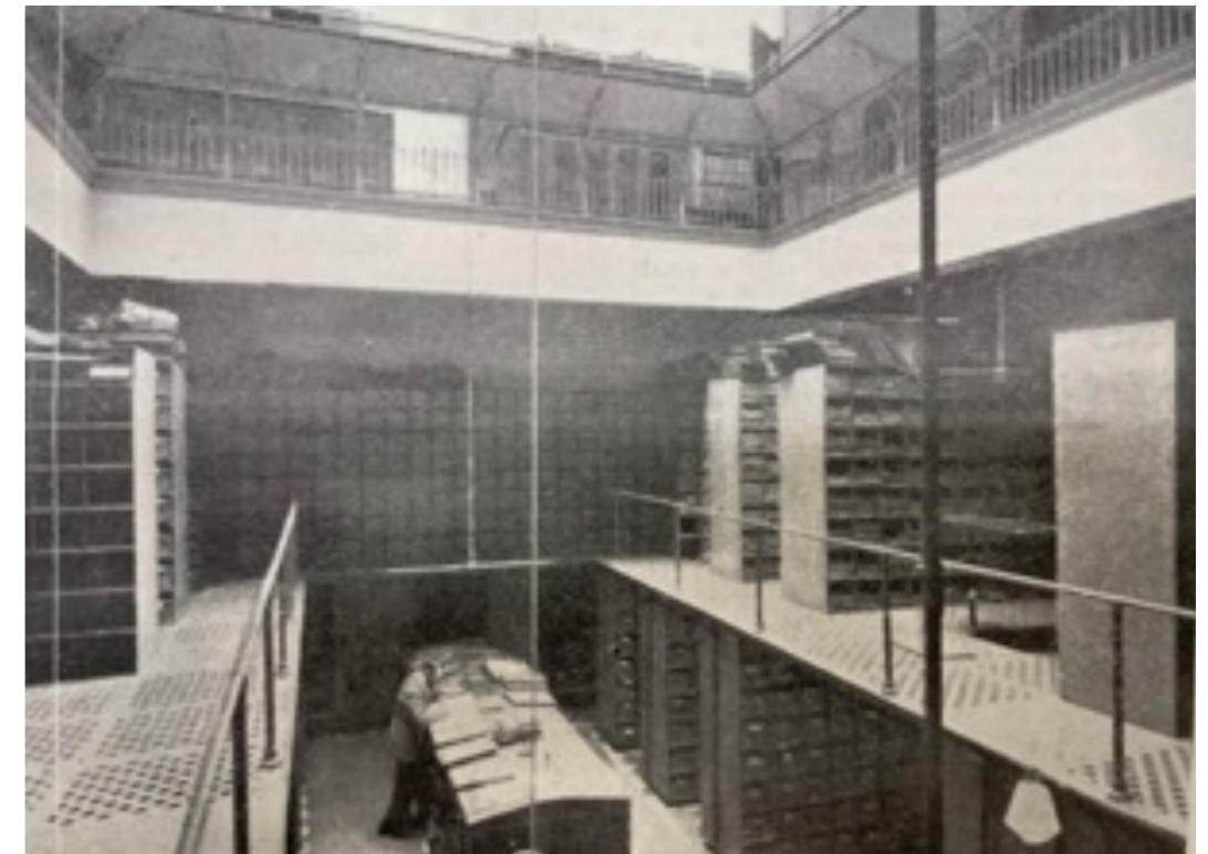
Lands Department building, Levels of the Strong Room with shelving, Town and Country Journal , January 1898.
