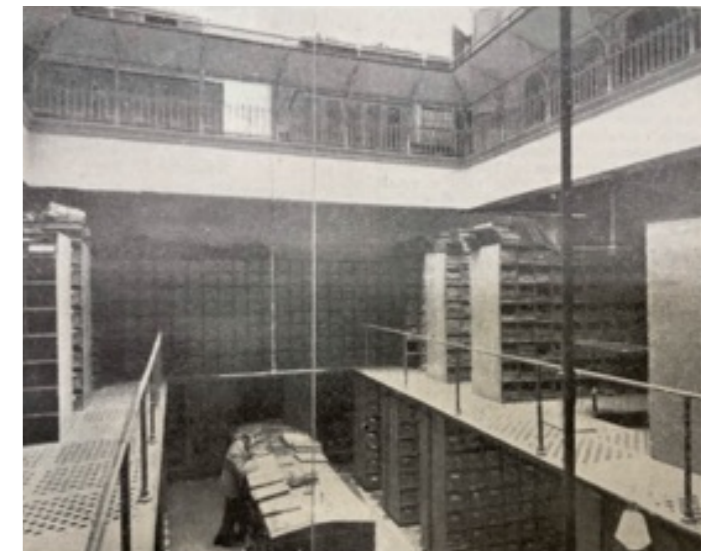
Lands Department building, Levels of the Strong Room with shelving, Town and Country Journal , January 1898.
