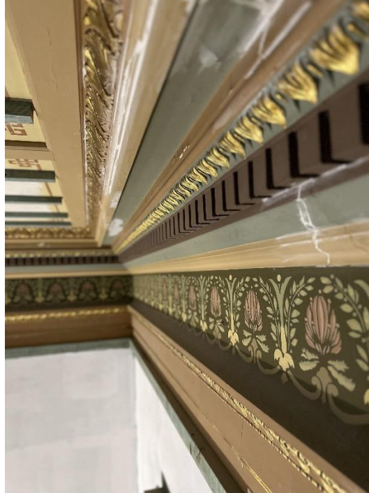
Plate 1: Detailed image of the ornate plaster cornice and string moulding in G.07
