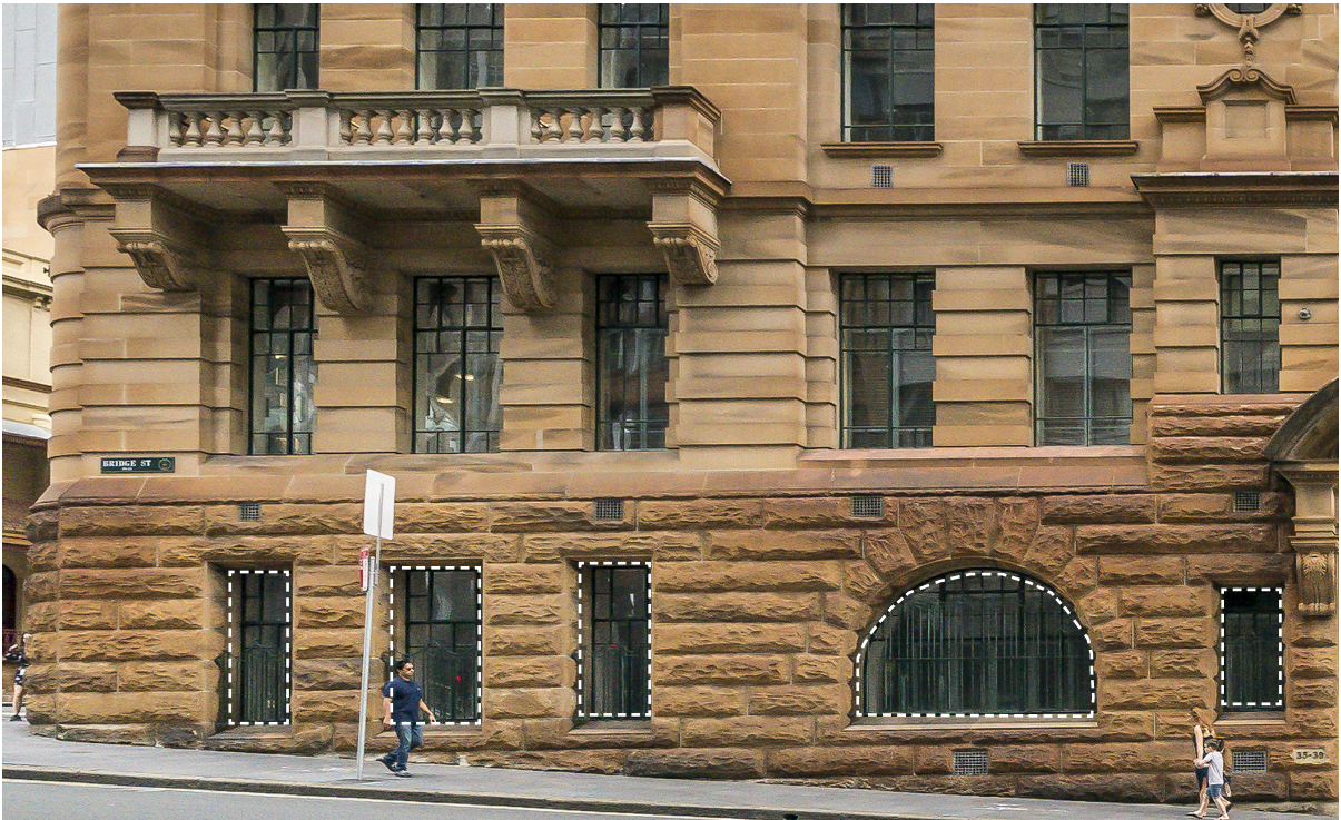
A: Bridge Street (North elevation)
