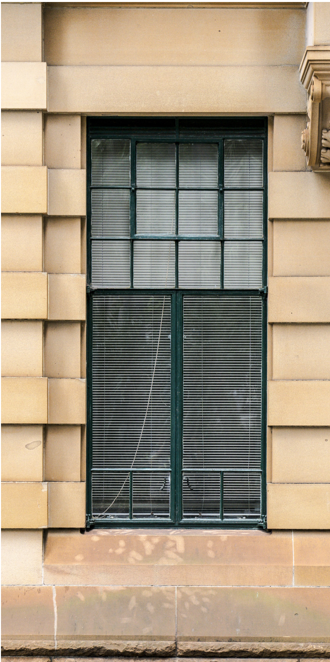
Existing window on Loftus Street (same type)
