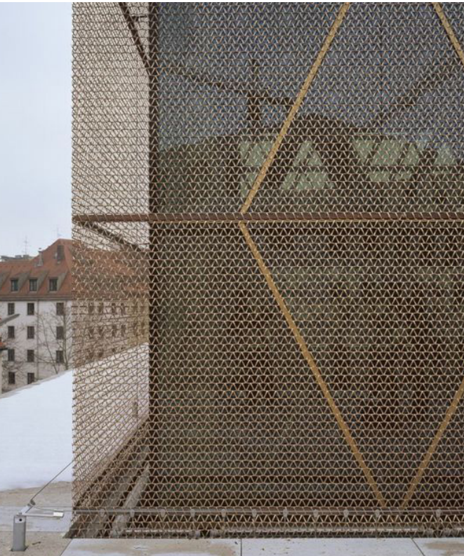
Existing screen above Farrer Place entrance (top), Paul Smith, 6a Architects (bottom)
