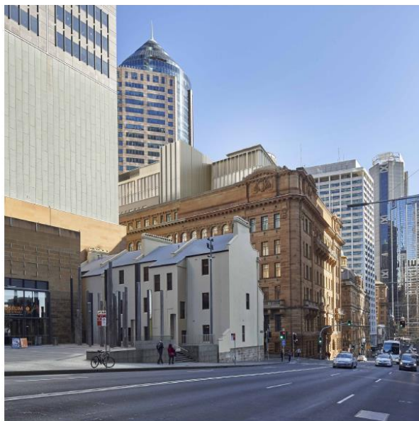
MOD 3 Bridge Street view
