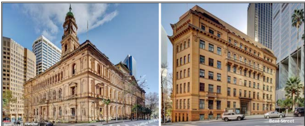
Figure 2 | View north-west to the Lands Building (left) and view north-east to the Education Building (right)
