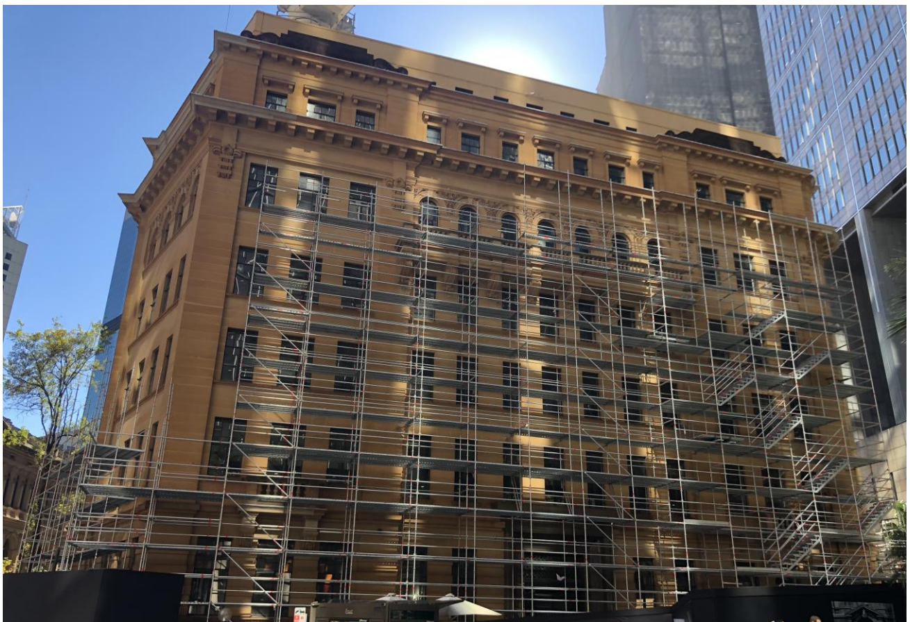
Figure 2 The Education Building viewed from Bent Street to the south
