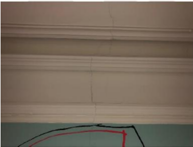
Typical hairline cracking through decorative cornice
