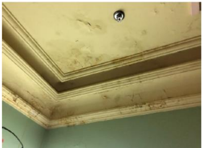
Moisture damage to timber lath and plaster ceiling
