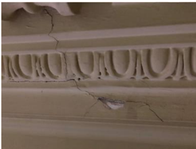
Typical cracking to decorative moulding, evidence of water damage present
