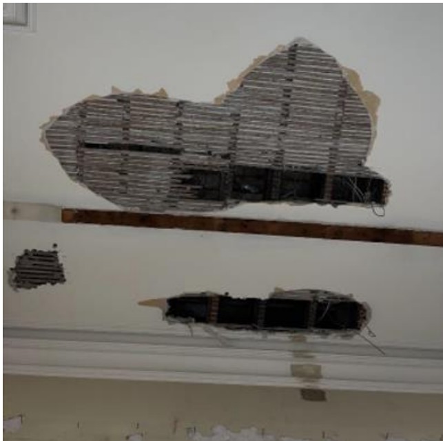
Typical example of collapsed timber lath and plaster ceiling
