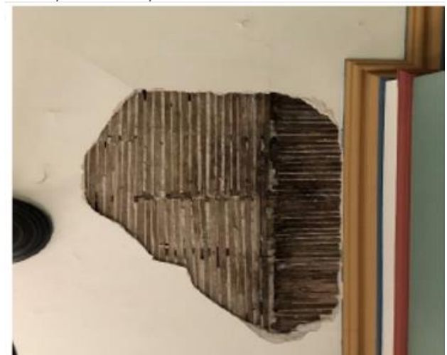
Ceiling collapse, discoloration of timber laths suggestive of moisture damage. Framing of laths appears to have changed here.
