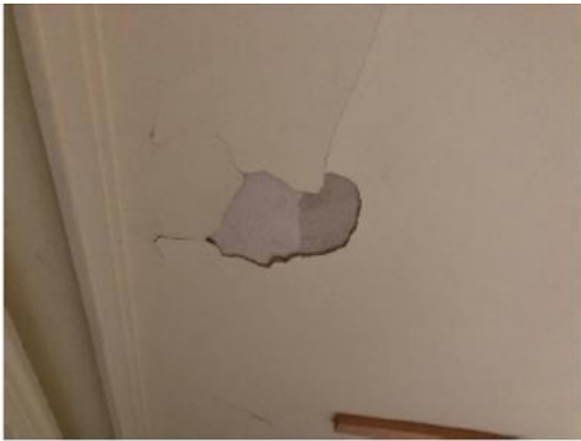
Typical example of separation of paint from plaster
