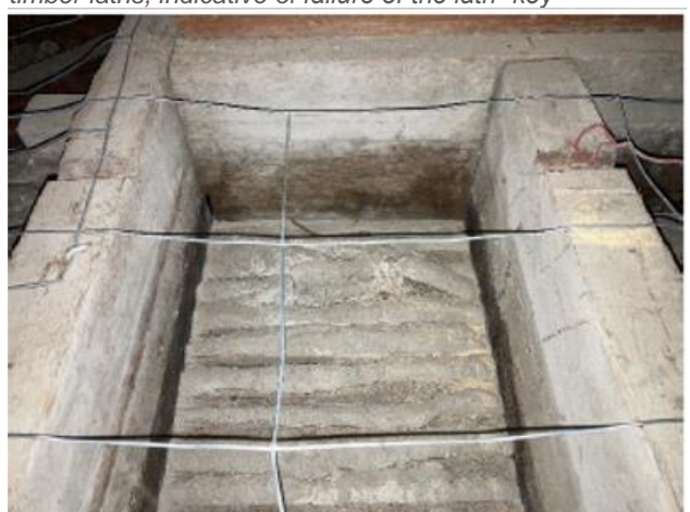
Example of broken key at timber lath ceiling
