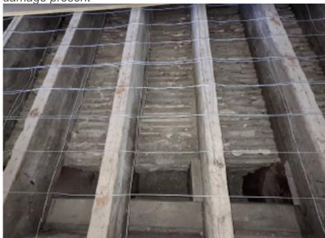
Example of missing keys at topside of timber lath ceiling
