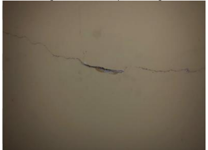
Full depth crack to plaster
