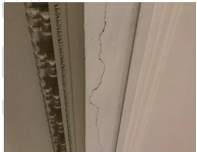
Typical cracking to the decorative moulding, parallel to the timber laths, indicative of failure of the lath "key"
