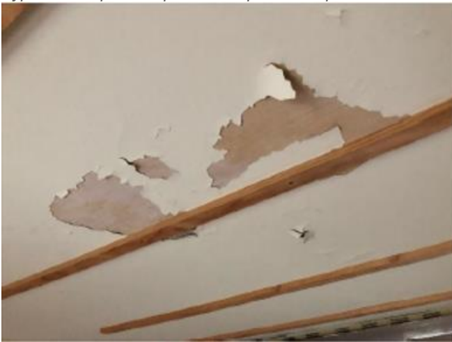
Typical photo of delaminating paint system
