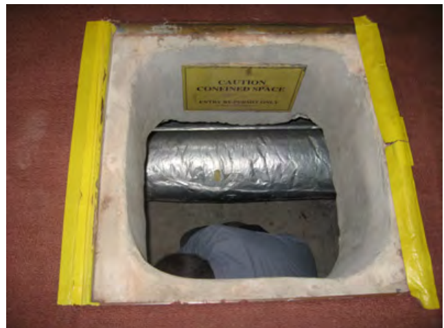
Figure 3.68 View into a service tunnel below the corridor floor
