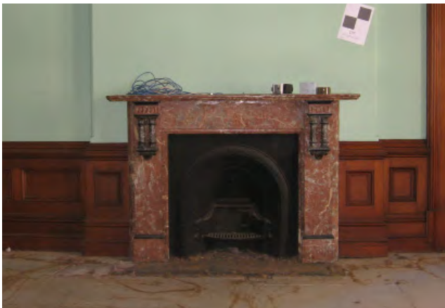
Figure 3.61 Fireplace in Room 207
