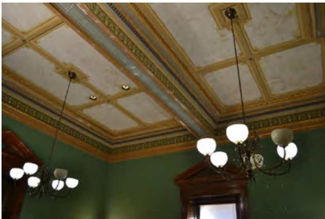
Figure 3.74 Ceiling of Room 107 currently being repaired
