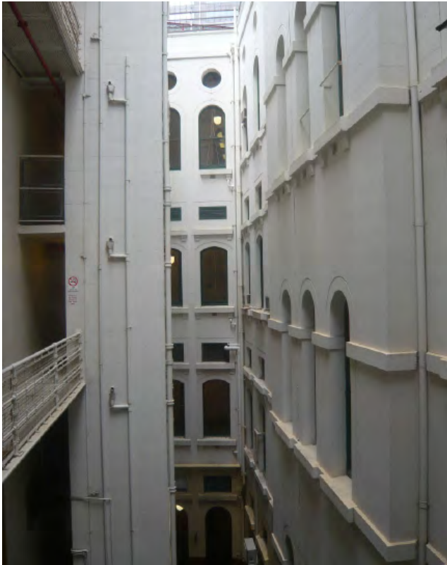
Figure 3.54 View of internal lightwell with suspended walkways to toilets
