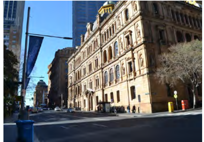
Figure 3.6 The Lands Building seen from the northwest side of Bridge Street
