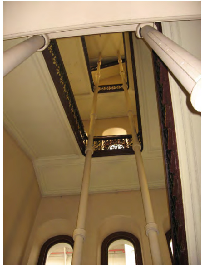
Figure 3.48 Stair shaft off Bent Street entrance
