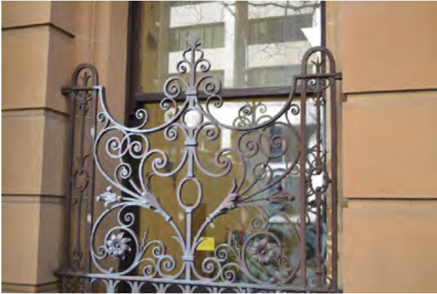
Figure 3.42 Typical wrought iron window grilles on ground floor level
