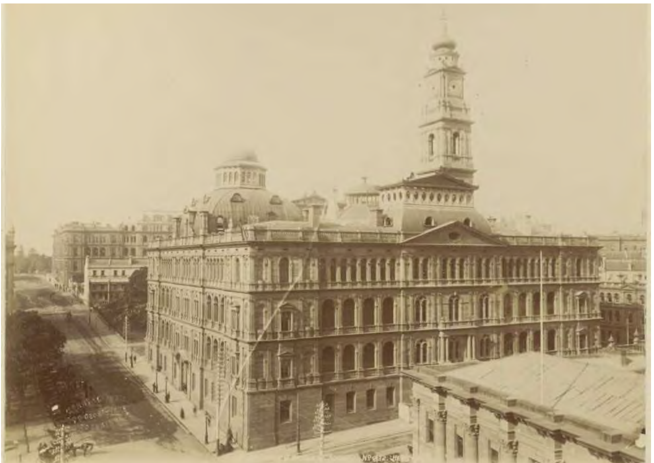
Figure 2.20 The Lands Building after the completion of the second stage, c1894, showing the Bridge and Gresham Street elevations Source: National Library of Australia, Call No. PIC/929/228 LOC Album Large Albums, nla.obj-138638327
