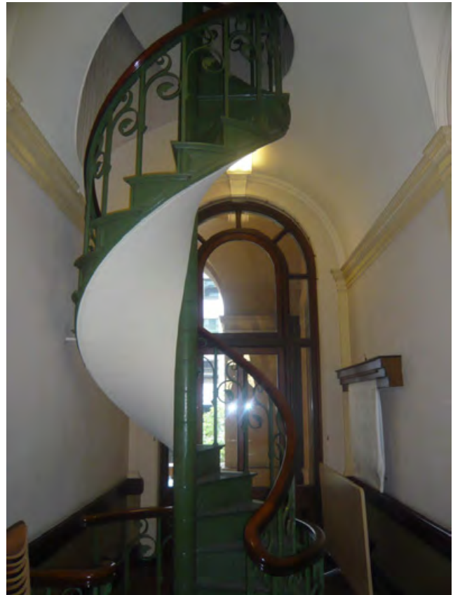
Figure 3.52 Cast iron spiral staircase between the ground floor and second floor
