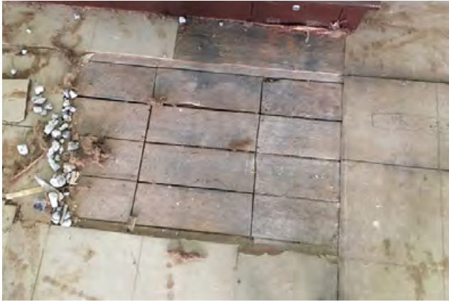
Figure 3.76 Saw cut timber floor boards
