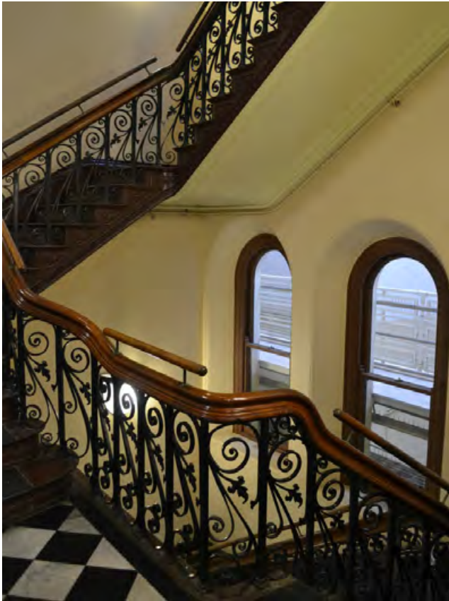
Figure 3.50 Stair off Loftus Street entrance
