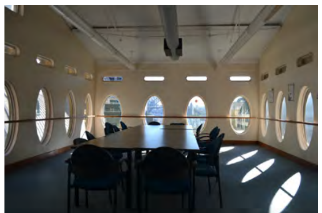
Figure 3.30 Internal view of the eastern pavilion (tempietto mansard) room. Glazing in all the metal framed windows has been replaced at some point in the recent past and, for the most part, has been fixed with silicone.
