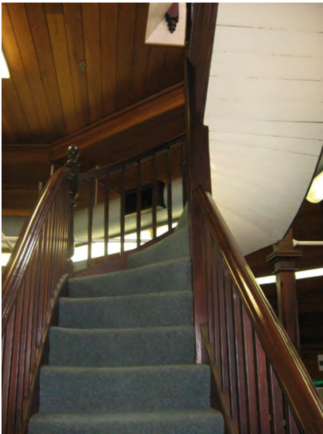
Figure 3.51 Timber stair in northern dome
