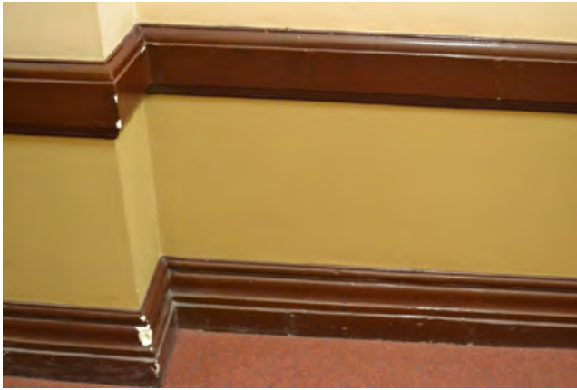
Figure 3.80 Corridor plaster skirting
