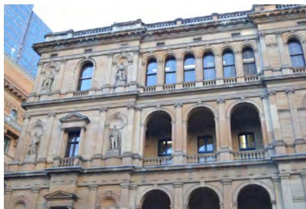
Figure 3.13 Arcaded verandahs and niches with statues on the Bridge Street elevation
