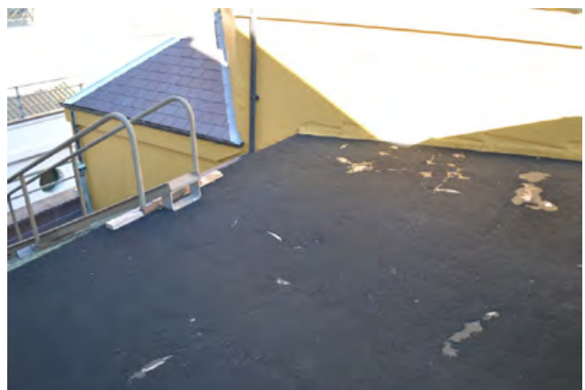
Figure 3.37 Detail of membrane roof adjacent to the east of the central strong room
