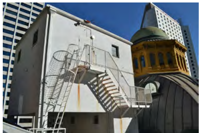
Figure 3.38 External view of the 1950s lift overrun and motor plant with steel walkways, ladder and stairs
