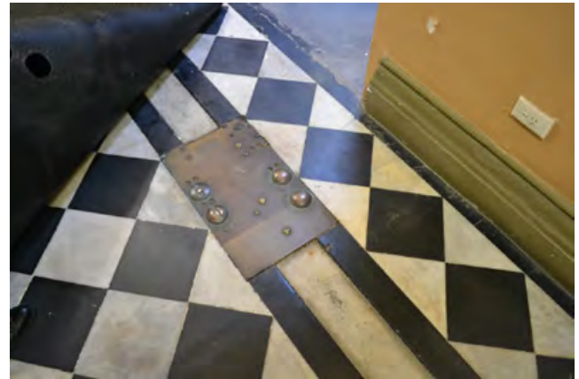
Figure 3.79 The surveyor's base line in the ground floor corridor
