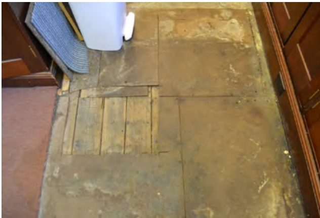
Figure 3.77 Timber floor boards under linoleum and carpet finishes
