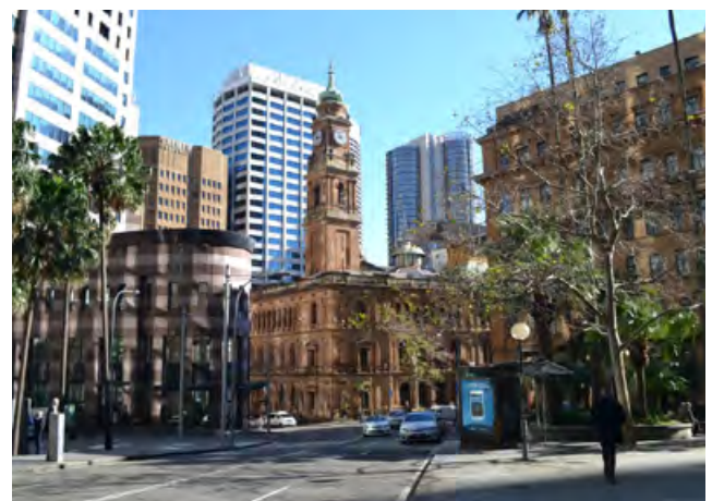
Figure 3.10 The Lands Building seen from Bent Street, with the Education Building and Farrer Place on the right
