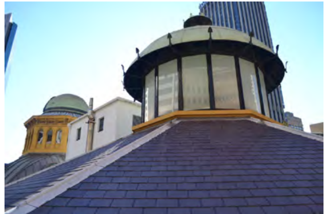
Figure 3.28 The central copper dome/lantern over the strong room
