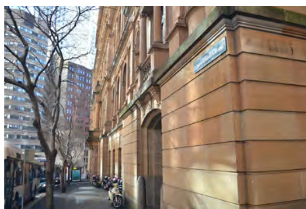
Figure 3.14 Rustication on the corner of Gresham and Bent Streets, looking north
