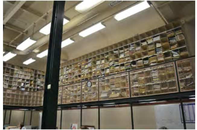
Figure 3.64 Internal view of the strong room, showing the cast iron mezzanine floor and catwalks
