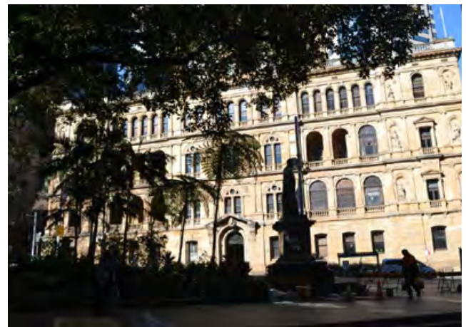
Figure 3.8 View of the Bridge Street elevation of the Lands Building as seen across Macquarie Place
