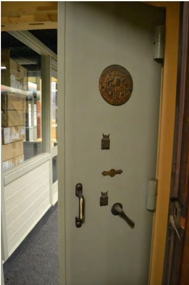
Figure 3.63 Milners 212 patented and improved fire and thief resisting doors to the strong room. The doors were manufactured by English firm Milners Safe Company, until 1874 known as Thomas Milner & Co.
