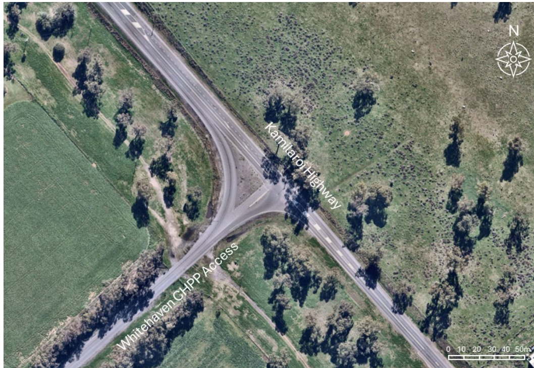
Figure 4.3: Whitehaven CHPP Intersection with Kamilaroi Highway
