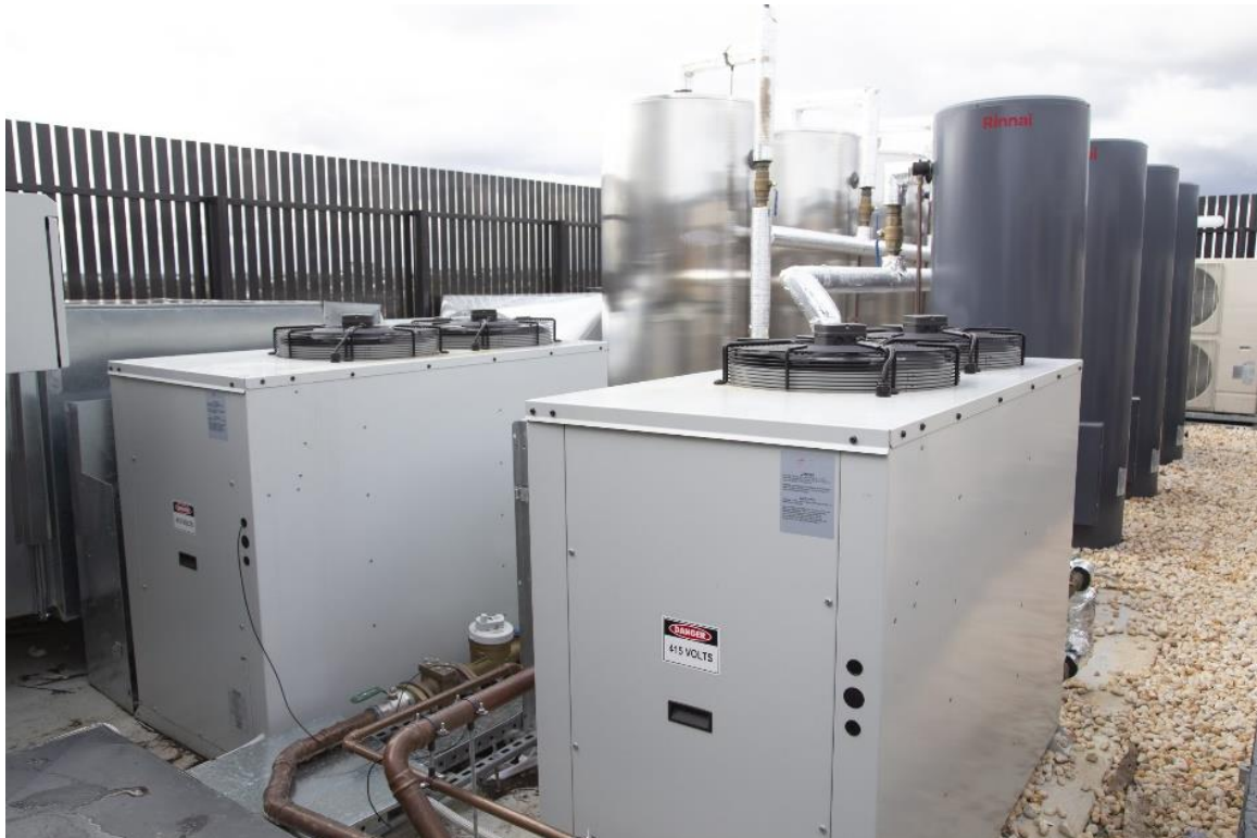
Figure 4- Typical heat pump set up
