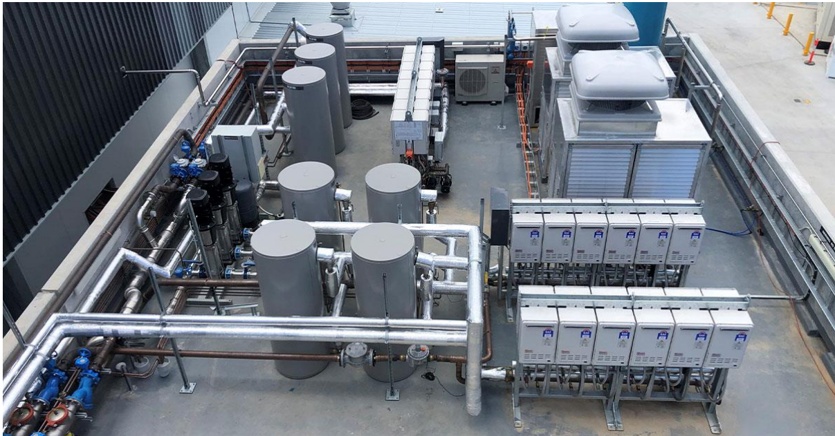
Figure 5 - typical gas hot water plant
