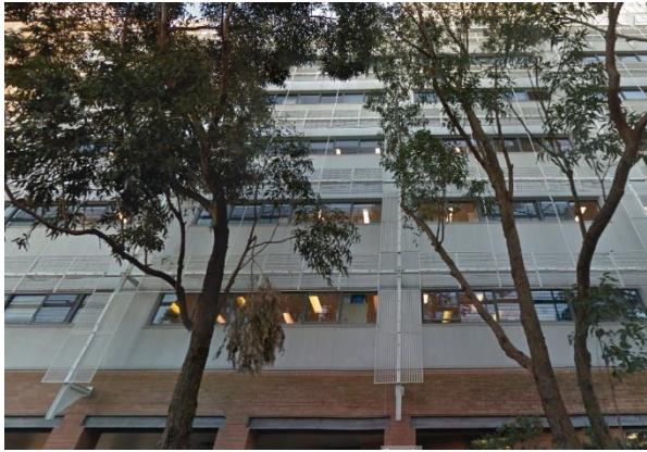
Figure 5 North View: Samuels Building (F25)
