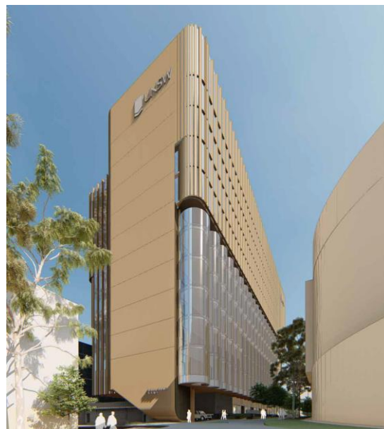
Figure 2 G25 Building view from G11 Botany Road
