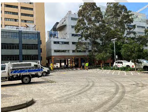
Figure 17 – Entry to carpark, facing north
