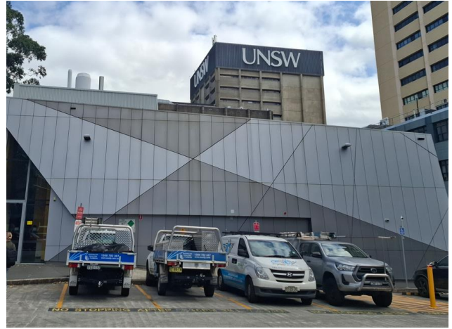
Figure 8 Exterior view of the Solar Industrial Research Facility (Building G23) facing west.
