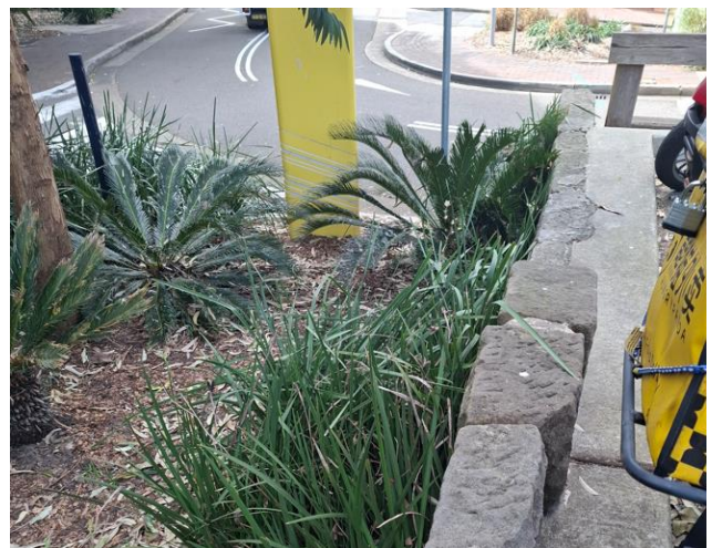
Figure 18 Exterior view of sandstone wall in the northeastern corner of parking lot and Gate 11 Avenue.
