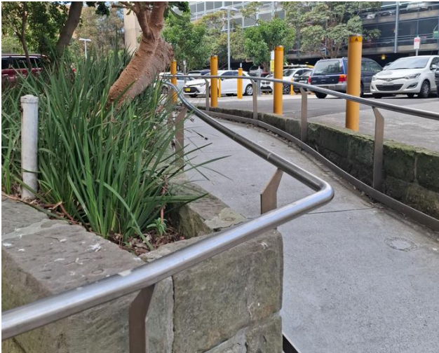
Figure 21 Exterior view of sandstone wall, metal railings and concrete wall, facing south-east.
