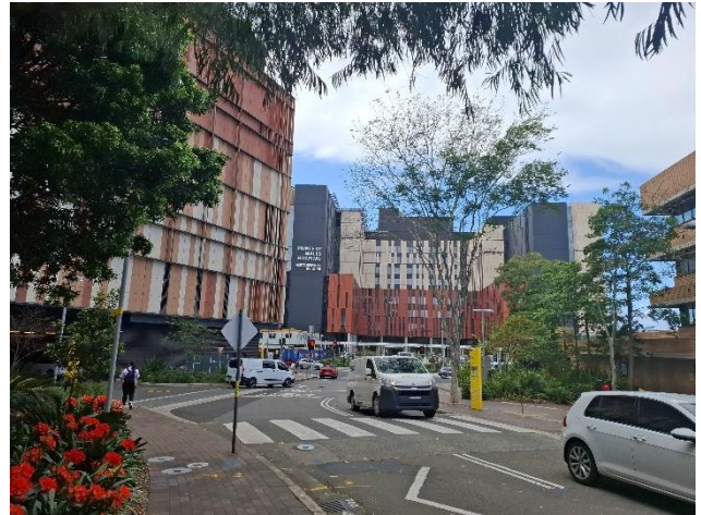
Figure 3 Exterior view to the Prince of Wales Hospital
