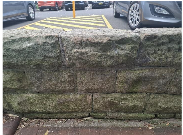
Figure 28 Exterior view of a close up of the sandstone wall, facing south.
