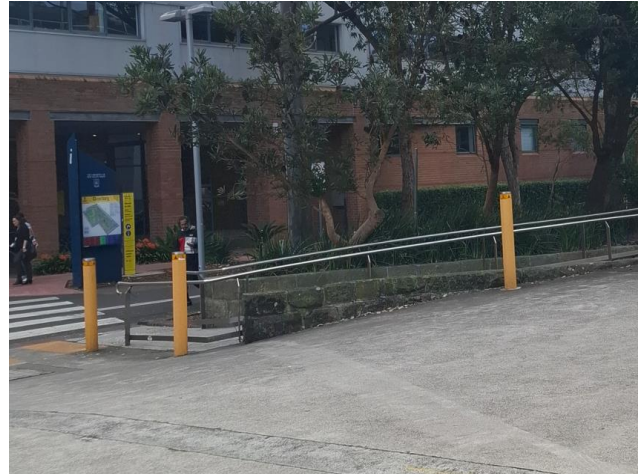
Figure 20 Exterior view from Building G23 to sandstone wall and concrete ramp, facing north east.
