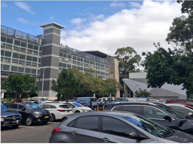
Figure 7 Exterior view of Botany Street Car Park (Building H25) facing south-west.
