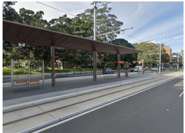
Figure 5 Exterior view of the UNSW Anzac Parade Light Rail
