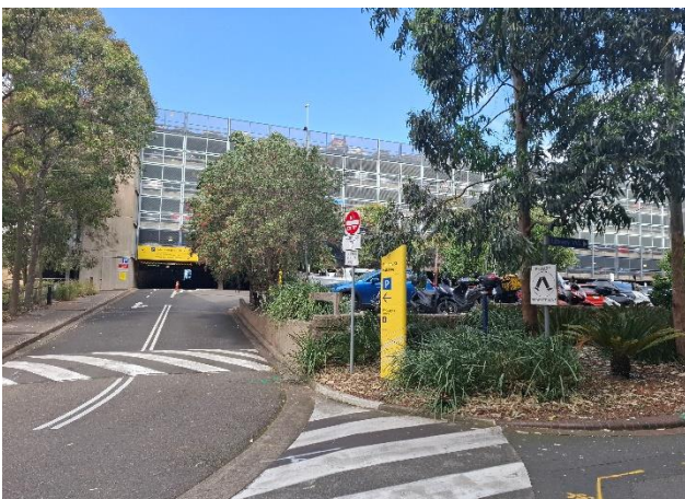
Figure 11 Exterior view of Gate Avenue 11, Building H25 and the sandstone wall, facing south.
