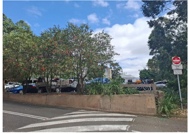
Figure 14 Exterior view from across the AGSM Building and the corner of the sandstone retaining wall, facing west.
