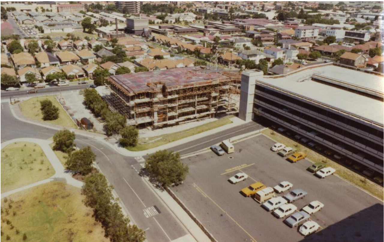
Figure 47 1979 photograph of the retaining wall and the newly built H25 Parking Lot.
