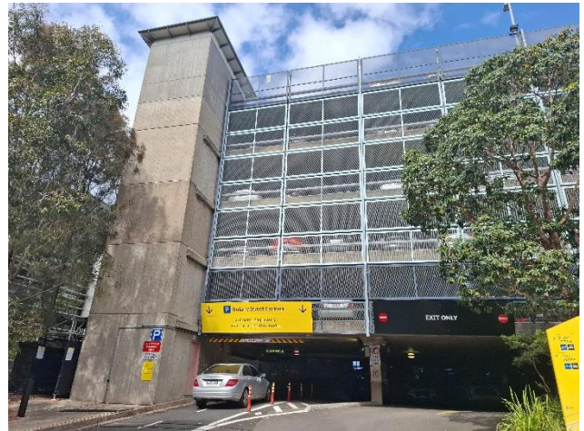
Figure 10 Exterior view of the Botany Street Car Park (Building H25) facing south.
