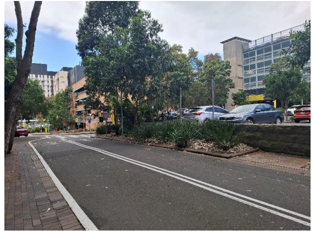
Figure 26 Exterior view of sandstone wall with Prince Wales Hospital and Building H25 in the foreground, facing south-east.
