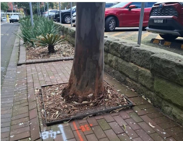
Figure 23 Exterior view of sandstone wall and pathway, facing east.
