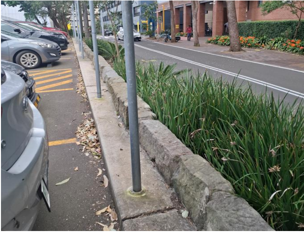
Figure 19 Exterior view of sandstone wall and library walk, facing west.
