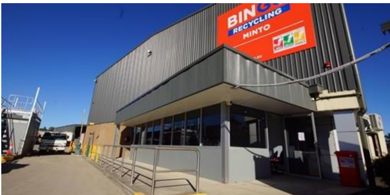
Plate 1: Exit weighbridge and existing office at Shed A
