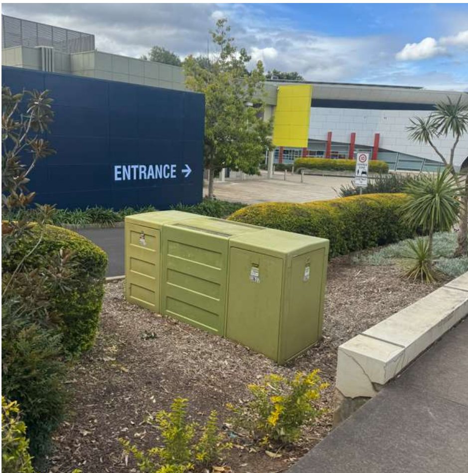
Image of S13617 on Site at Entry
