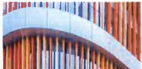
1. Concrete or aluminium facing to slab edges
