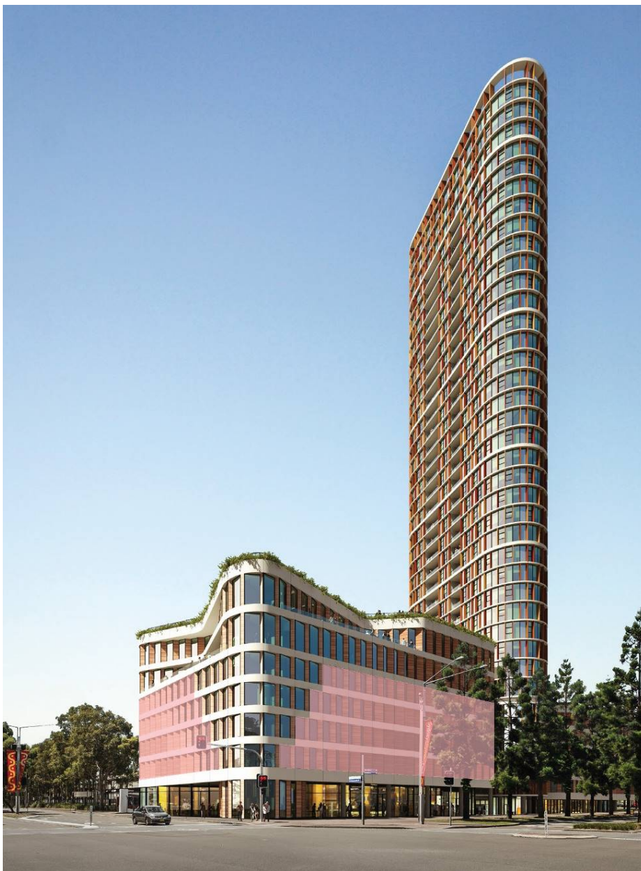
Figure 12 – Pink shading showing location of car park ventilation panels Source: Bates Smart
