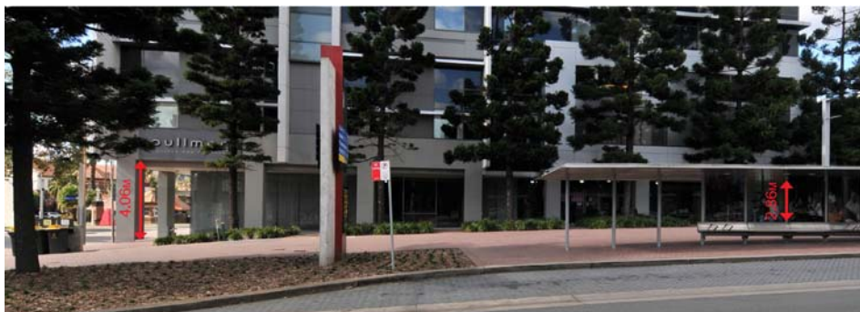
Figure 1 – Pullman Hotel colonnade, with height varying from 2.86 to 4.06 metres Source: Bates Smart
