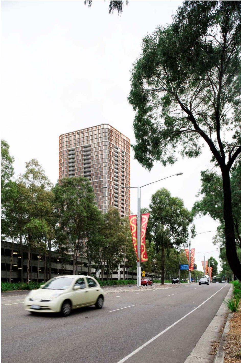
Figure 20 – Proposed development as viewed from Sarah Durack Avenue, with the P3 carpark in the foreground Source: Bates Smart
