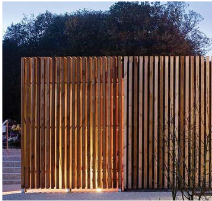
Timber Cladding to Garden Pavilions
