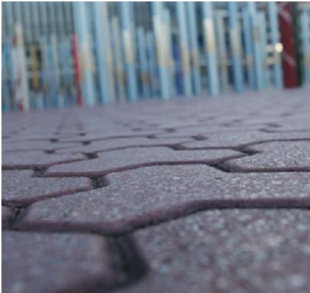
Trihex interlocking unit paving to match existing. Installed in accordance with SOP UEDM Section 3.1 Pavements.
