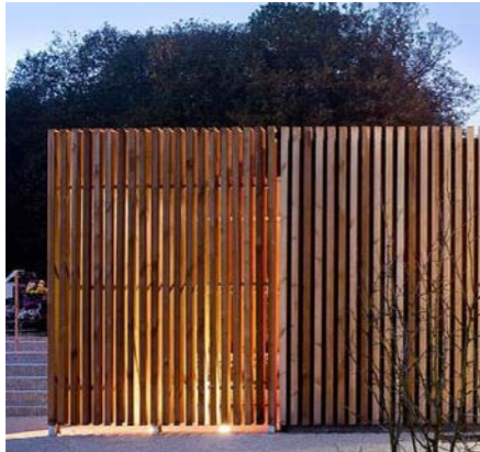
Timber Cladding to Garden Pavilions
