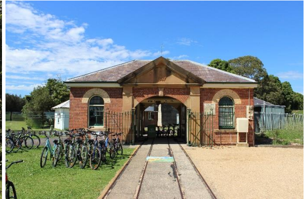
Figure 24: Entrance building to Millennium Parklands, showing light rail tracks, south aspect
