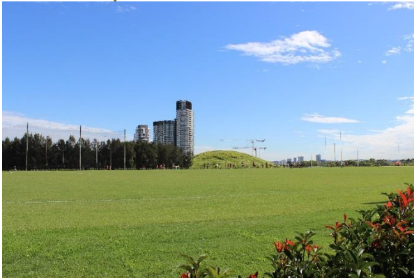
Figure 21: Australia Avenue Apartment complexes viewed from the Tom Wills Oval, northeast aspect
