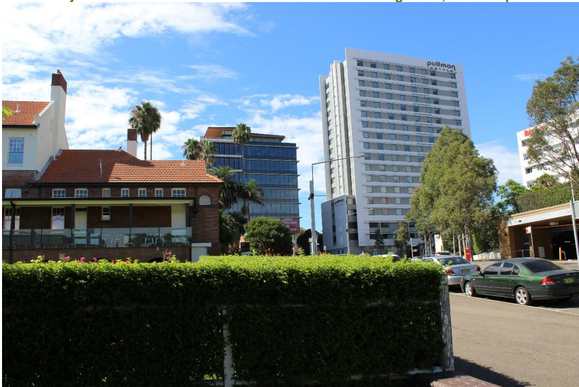
Figure 37: View of area of proposed development from Abattoir Heritage Precinct. Pullman Hotel and adjacent structures on Elliot Herb Avenue in the foreground, south aspect
