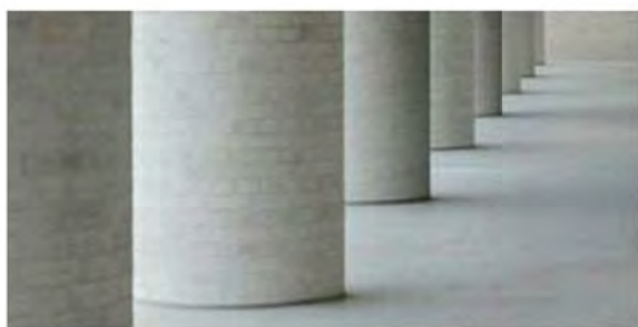
9. In situ concrete
