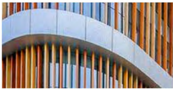
1. Concrete or aluminium facing to slab edges
