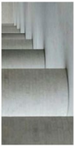
9. In situ concrete
