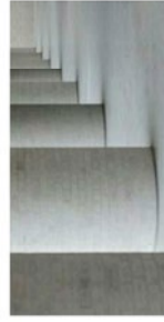
9. In situ concrete
