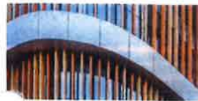
1. Concrete or aluminium facing to slab edges
