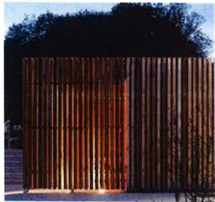
Timber Cladding to Garden Pavilions
