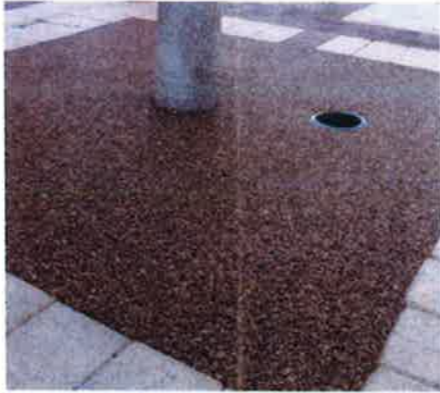
Tree Surround - 2.1m x 2.1m (Tree 1 only) Resin Bonded Porous Paving. Colour to match adjacent trihex paving. Required to retain tree and ensure clear movement around commercial lobby.
