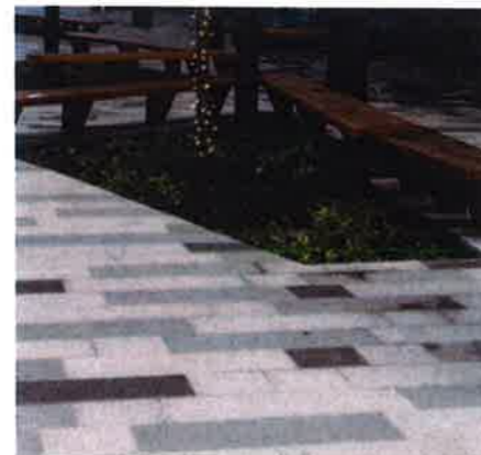
Flush planting and unit paving on structure
