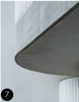
Concrete slab edge/ soffit
