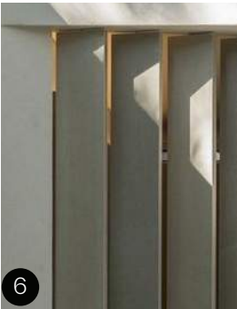
Concrete finished fin elements
