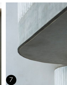
Concrete slab edge/ soffit
