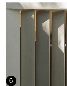
Concrete finished fin elements
