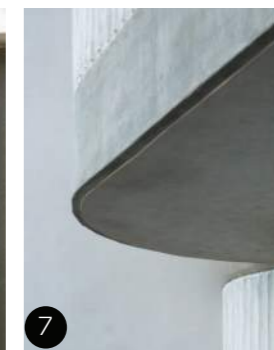
Concrete slab edge/ soffit
