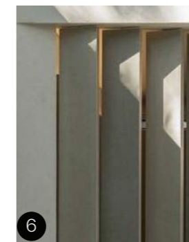
Concrete finished fin elements
