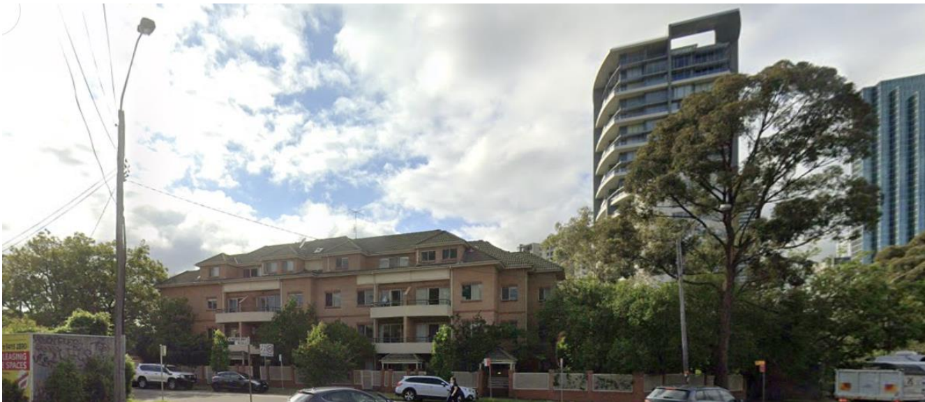
Site Context Photo - 849 - 859 Pacific Highway, and 2 and 8 Wilson Street, Chatswood
