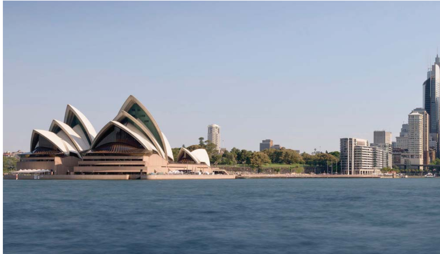
1. View from North Shore - Existing Ben Guthrie Photography
