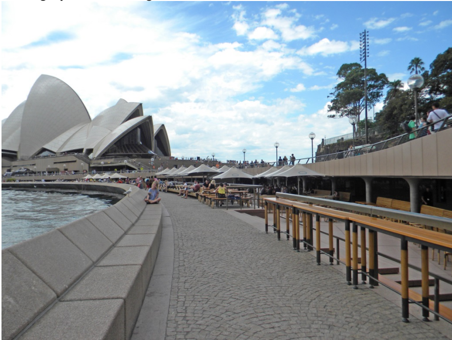
Photograph 2 – Existing Lower Concourse: View to the North
