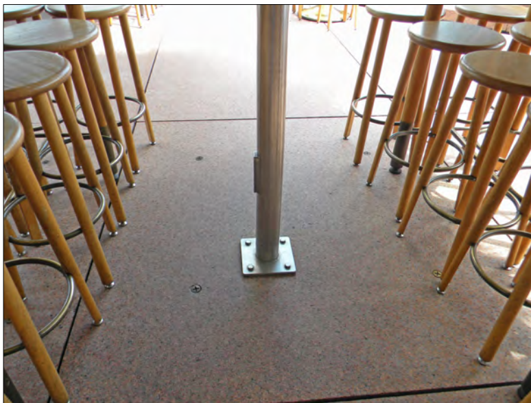
Figure 8: Showing how the existing umbrellas are anchored into the granite paving.
